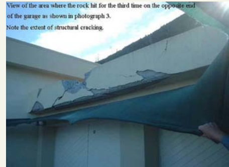
View of the area where the rock hit for the third time. Note the effect of structural cracking
