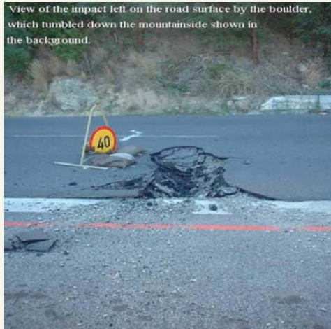
View of the road surface damage from a boulder that tumbled down the mountainside
