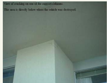
View of cracking on one of the support columns. This area is directly below where the vehicle was destroyed.
