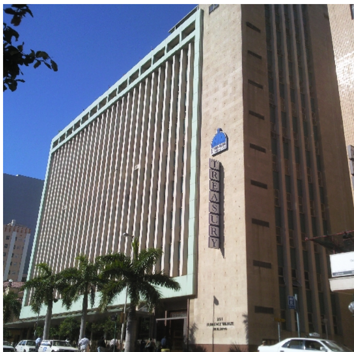
UNFAIR: Durban's municipal revenue treasury is at the Florence Mkhize building in Anton Lembede (Smith) Street.
