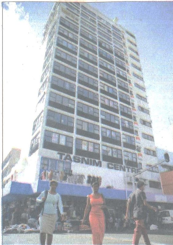
The face of Tasnim Centre after the wrap-around KFC advert was taken off the building.
